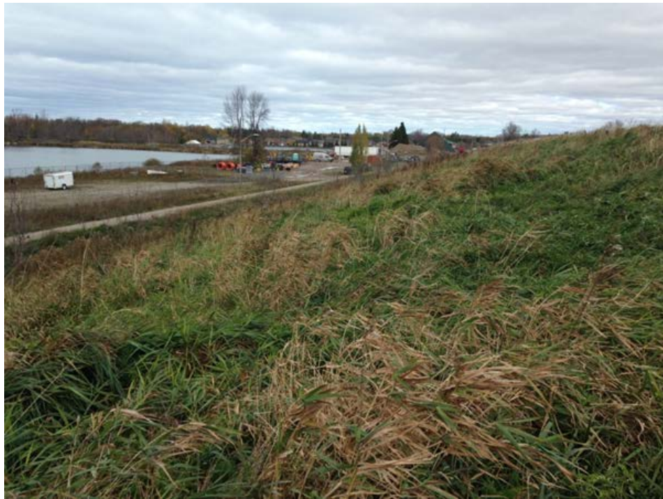
Photo 1 – West sideslope vegetation growth from southwest corner, looking north
