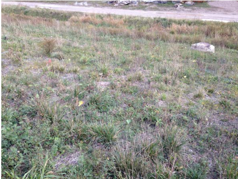
Photo 5 – Strong vegetation growth on repair areas on east sideslope
