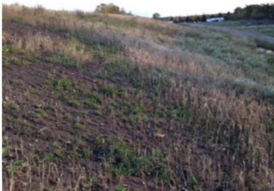
Photo 2 – Southeast corner manhole looking north lighter vegetation growth on the west side of the manhole with no signs of erosion
