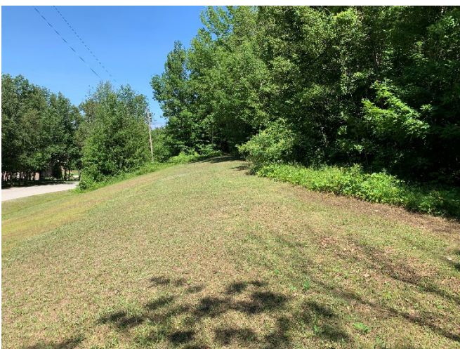
Photo 7: View of Kinhuron Road road-cut bank, facing northwest
